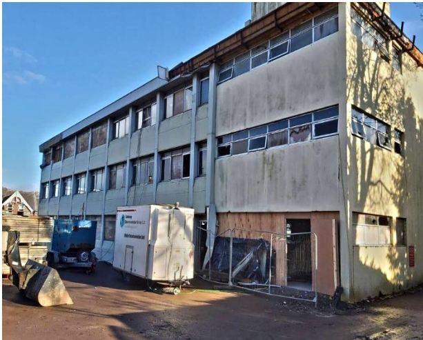
Springville House before the office-to-residential conversion
