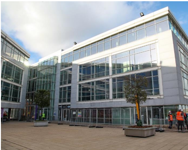
Park West Plaza before the office-to-residential conversion
